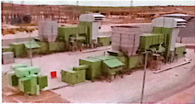
Rehab Gas Power Station (Frame 9E Gas Turbines)
