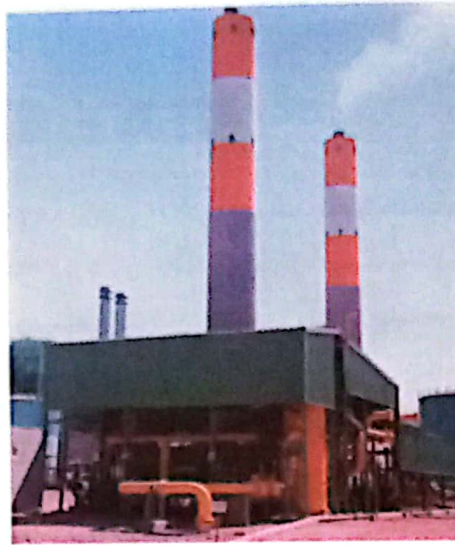
Aqaba Thermal Power Station Boiler Conversion to Dual Firing
