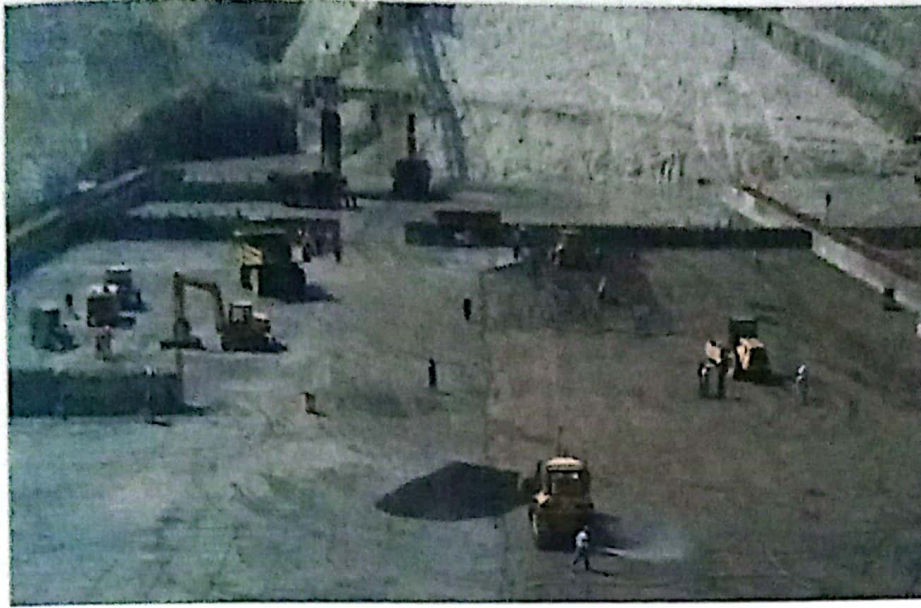
Equipment's Hauling, spreading & compacting the RCC
