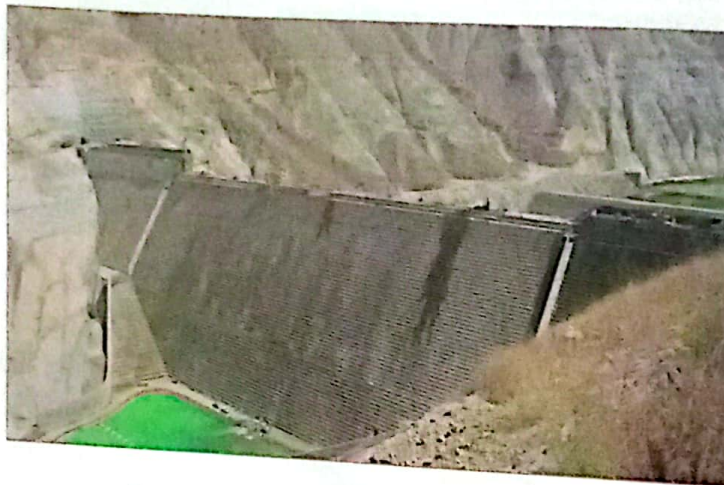
Alwehda Dam- Looking from Downstream
