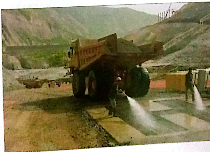
Cleaning for any equipment entering the RCC area
