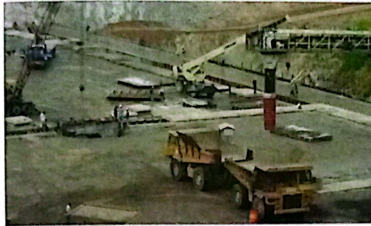
RCC Construction and Audit Gallery
