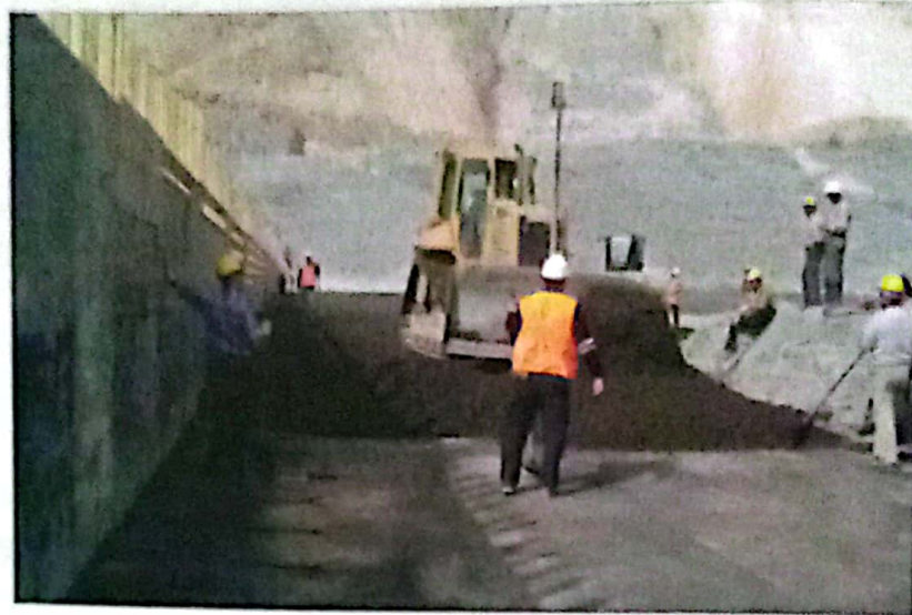
Spreading the RCC using Doze
