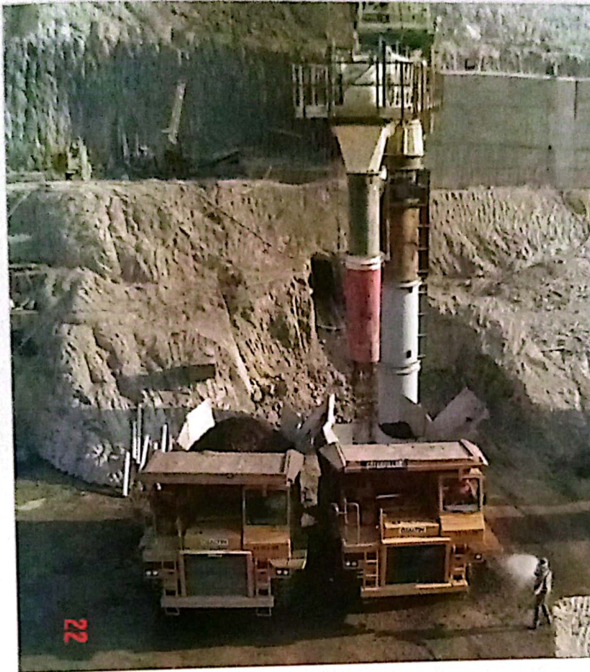
RCC Delivery using Conveyor belt and Vehicle
