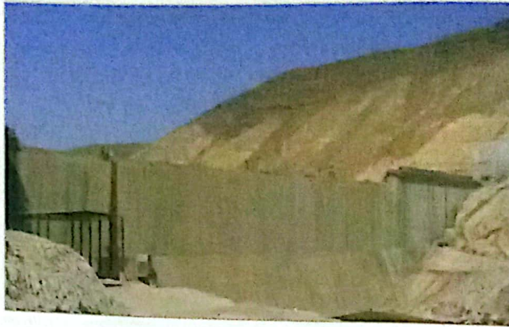
Alwehda Dam- Looking from Upstream
