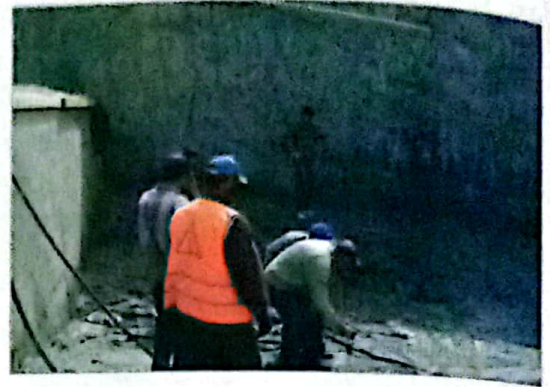
Preparation for foundation
