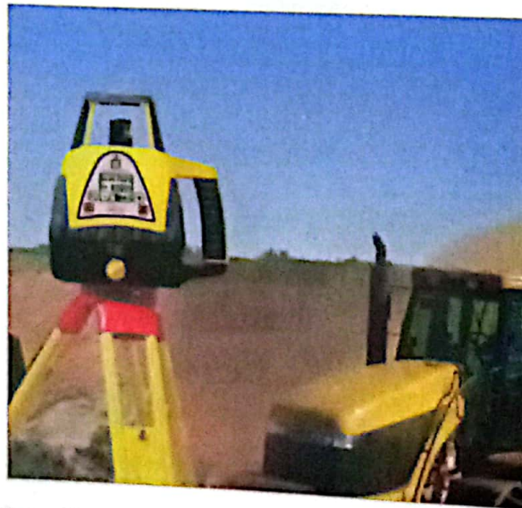
Laser Equipment Guiding Dozer during construction
