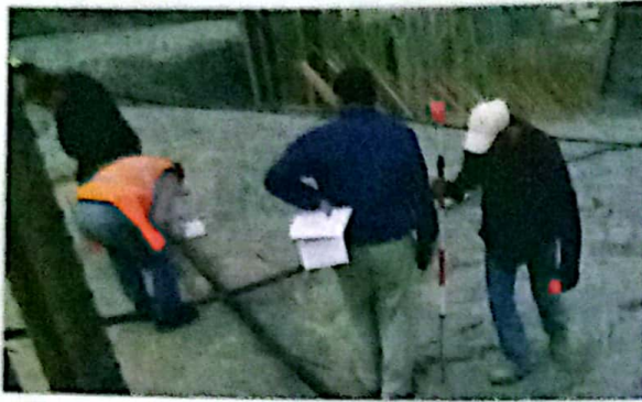
Inspection of foundation & Survey works for NGL
