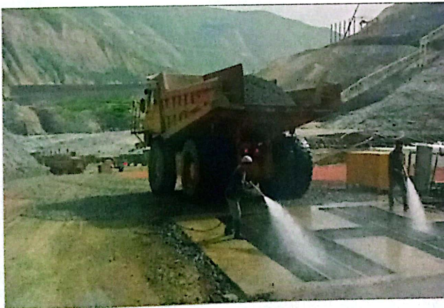
Curing of fresh RCC using mobile sprinklers
