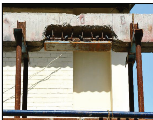
(b) Embedding the base plate at the mid-centre of the RC beam
