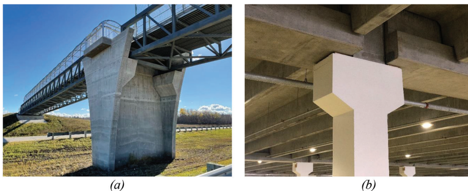
Fig. 1—Common applications of concrete corbels: (a) bridge pier bearing seat (single corbel); and (b) parking structure (double corbel).
