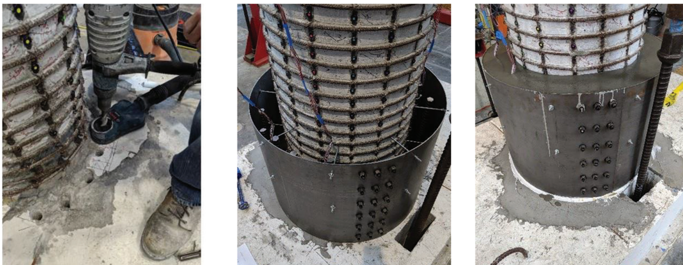
Fig. 4—Repair construction: (a) drilling holes; (b) assembling jacket; and (c) placing grout.
