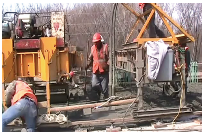
Fig. 2—Construction workers walking in previously vibrated concrete and causing loss in consolidation during construction of LC-HPC-12 Placement 1 (direction of placement is from left to right in picture).
